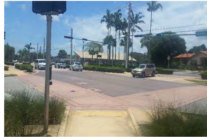
Old Cutler Road and Franjo Road: Brick Pavers and Stamped Asphalt Crosswalk were constructed as a part of a previous study which allow better access and safety for pedestrians.
