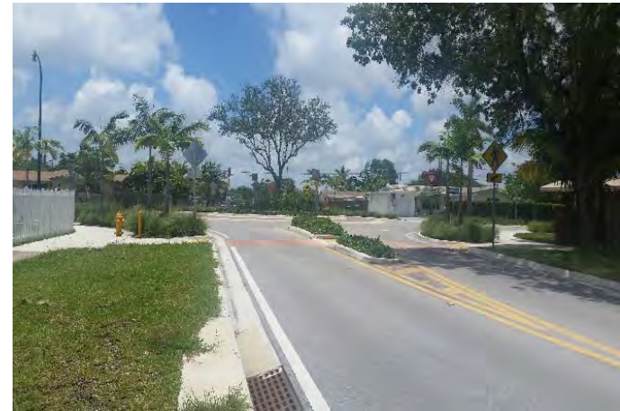
Caribbean Boulevard and Gulfstream Road: Roundabout was constructed as a part of the Town's previous studies to encourage vehicles to slow down and reduce crashes.
