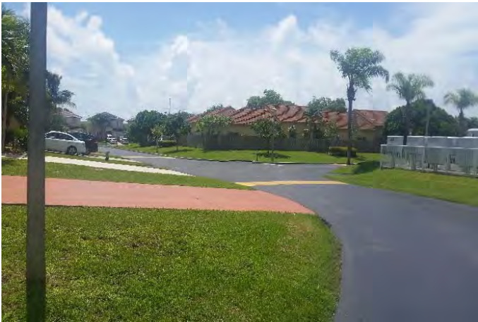
SW 87 Place and SW 214 Lane: Speed Bump was observed at this location. This type of device is placed to slow down motor vehicle traffic in order to improve safety conditions within the residential community.
