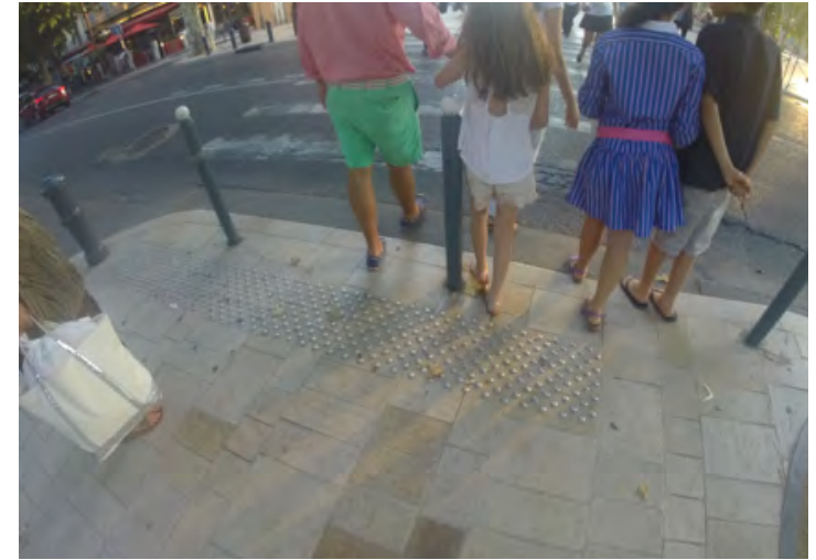
Barriers and changes in pavement texture create safer crossings.
