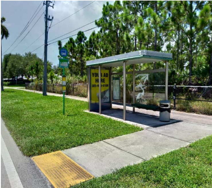
Figure 41: Photo of Existing Bus Shelter at SW 87 Ave, west side
