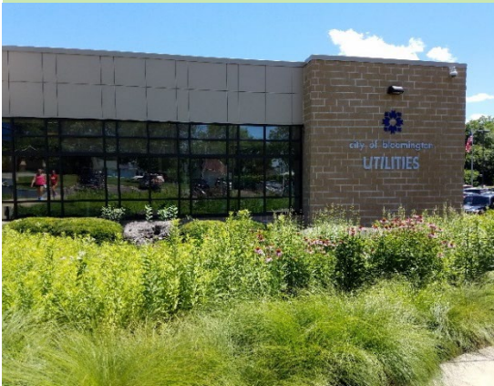
Figure 4.2.1. Rain Gardens can be designed to blend with a building's landscaping.
