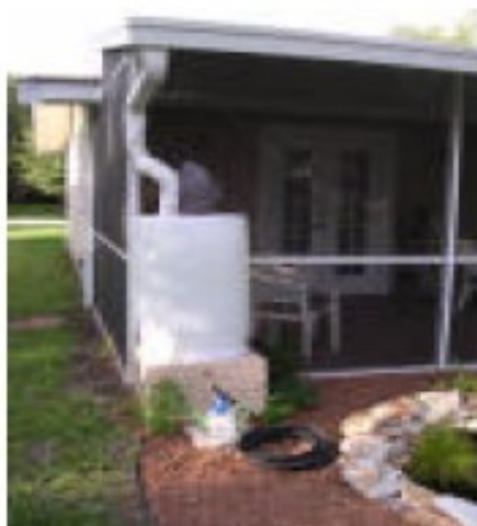
Figure 4.6.3: Type 1: Rainwater Harvesting with a Rain Barrel
