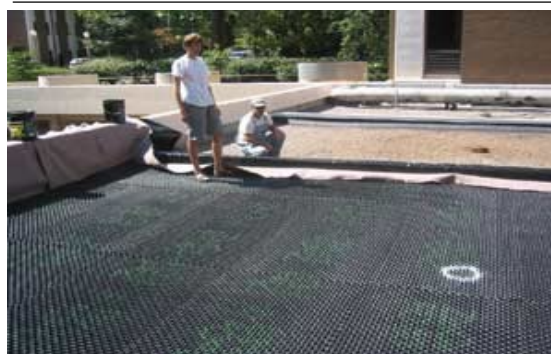
Figure 4.7.5. Drainage Layer Installation
