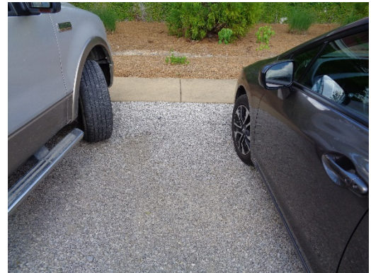
Figure 4.4.2. Permeable Pavement installed in a parking lot application
