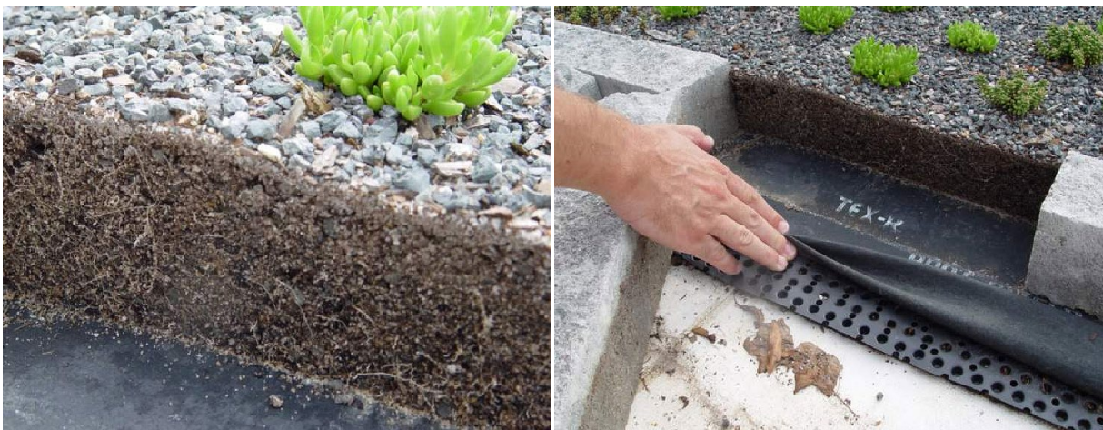
Figure 4.7.3. Greenroof Cross-Sections
