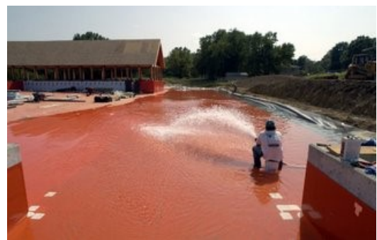
Figure 4.7.4. Flood Testing the Waterproofing Layer
