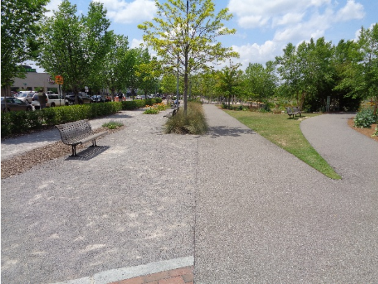
Figure 4.4.1. Permeable Pavement incorporated into sidewalk design
