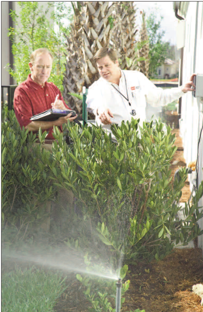
Simple steps, such as checking the alignment of sprinkler heads, can improve the efficiency of automatic irrigation systems and ensure the right amount of water goes where it is needed.
