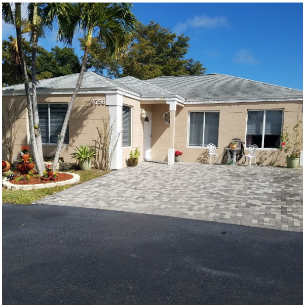
Property elevated on fill above street
