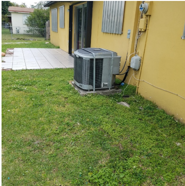
HVAC secured at grade
