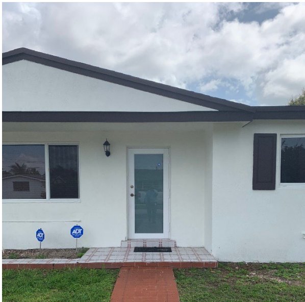
Property elevated 8" above grade
