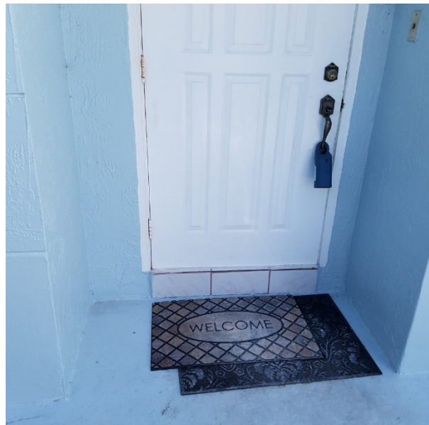
Home elevated approximately 8" above grade
