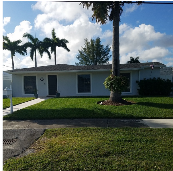
Home elevated approximately 8" above grade; storm drain in front of house
