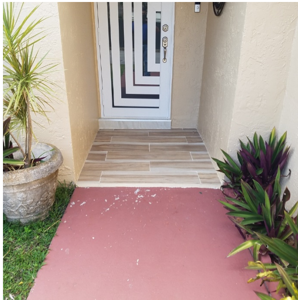
Finished floor elevated above grade
