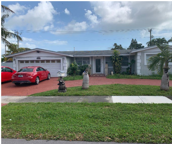
Property elevated about 1 foot above street
