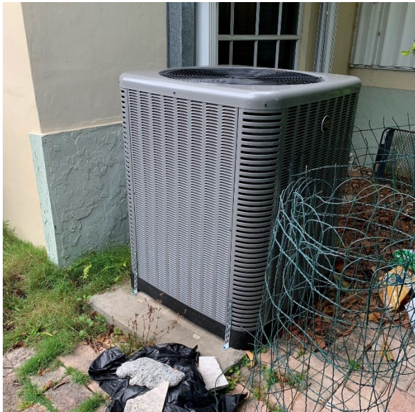
HVAC secured at grade
