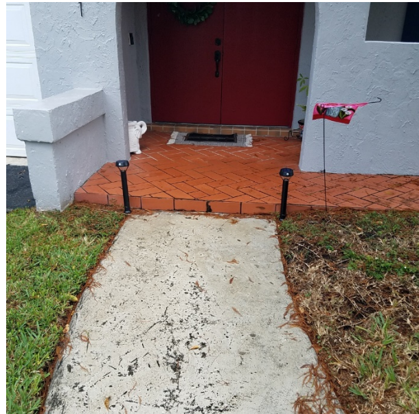
Home elevated approximately 8" above grade
