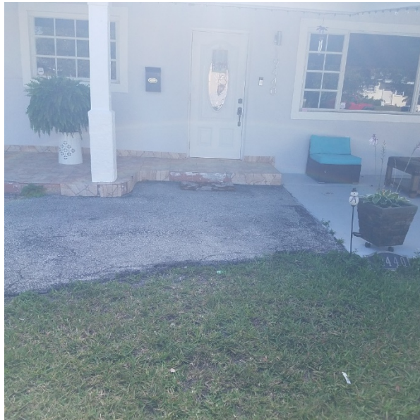
Property elevated approximately 10" above grade
