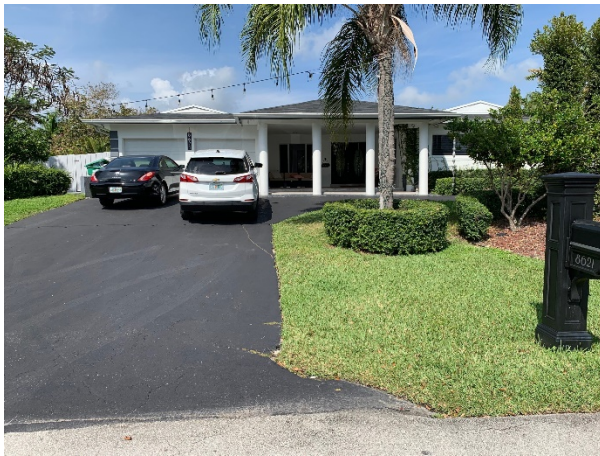
Property elevated on fill approximately 42" above street level
