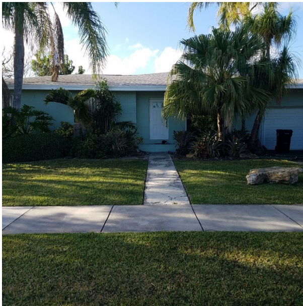
Property elevated on fill above street
