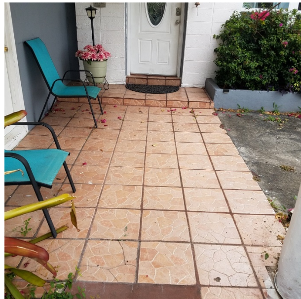
Finished floor elevated approximately 10" above grade
