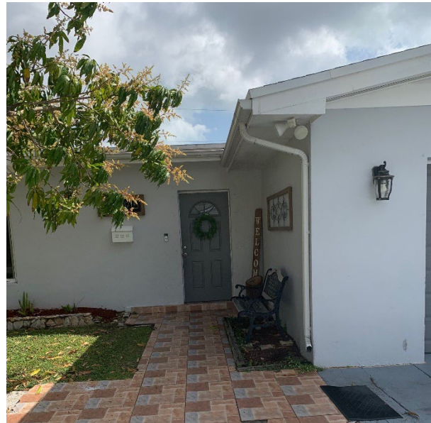
Guttering drains to driveway
