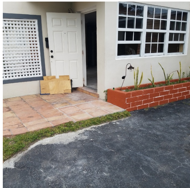
Home elevated approximately 8" above grade
