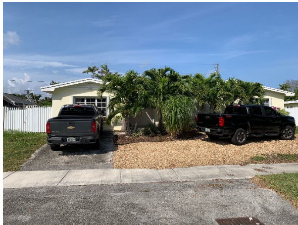
Storm drain in front of property
