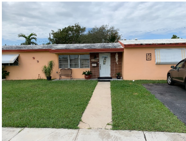
Property elevated on fill above street
