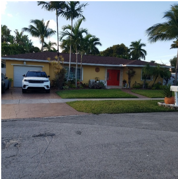
Property elevated on fill above street, home elevated above grade
