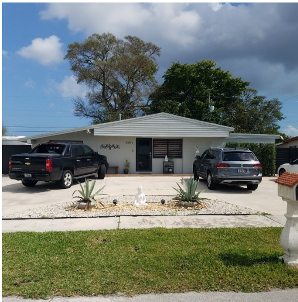
Driveway/Parking pad creates large amount of impervious surface
