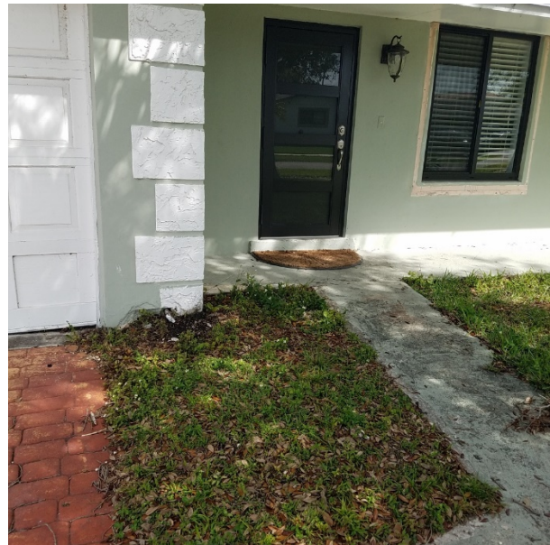
Home elevated approximately 6" above grade
