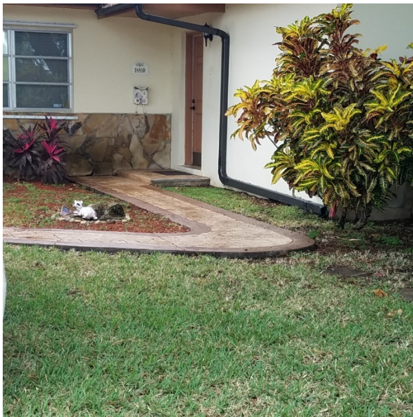
Property elevated 8" above grade, guttering drains to front yard at foundation
