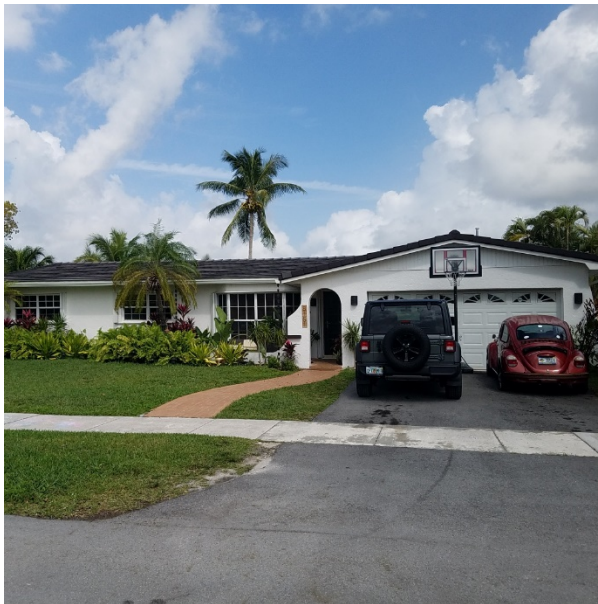
Guttering drains to front garden bed; slight grading away from house
