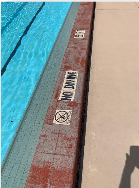
Depth and warning tiles in gutter coping
