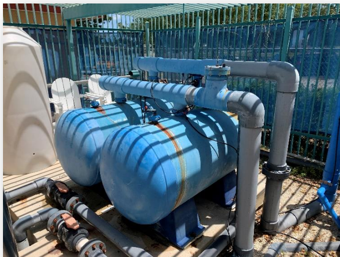
Horizontal sand filters with inflow and effluent lines
