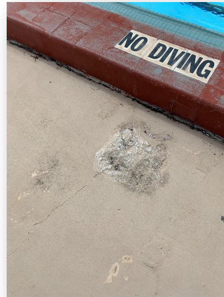
Concrete spall on north side
