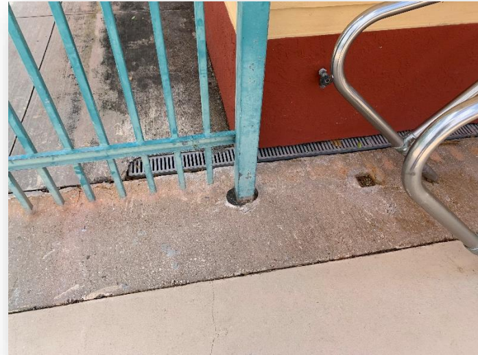
Deck drain settlement and separation at concession building
