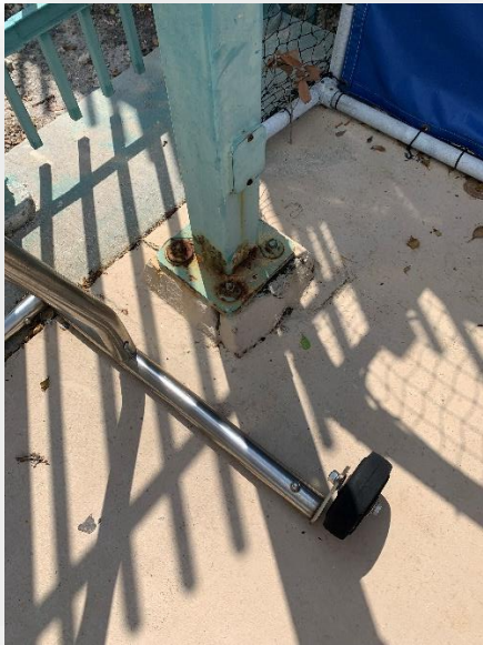
Light pole base showing corrosion in SE corner
