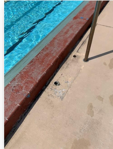
Old ladder inserts sticking up from deck
