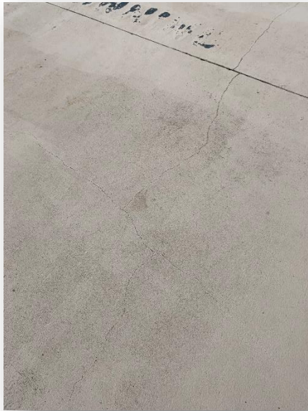
Shrinkage cracking in deck on north side
