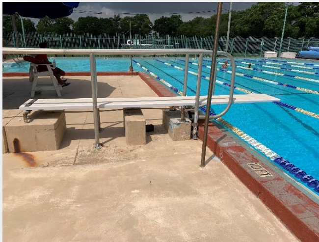
Cracks, rust, and corrosion on dive pedestals
