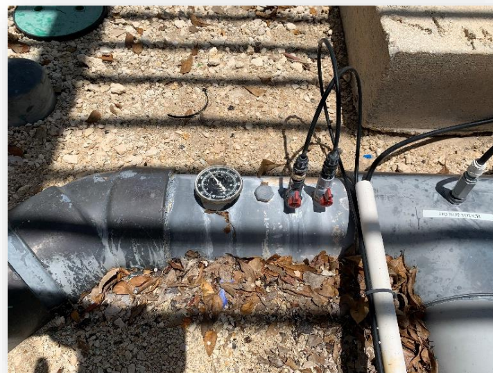
Chemical feed injection points
