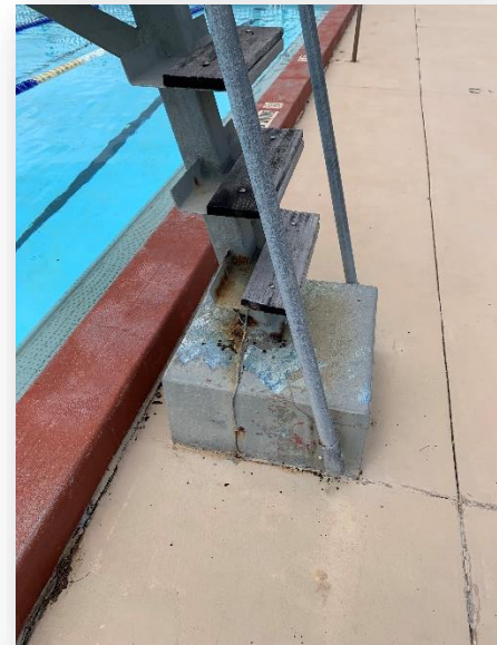
Lifeguard stand on north side showing distress and exposed wire
