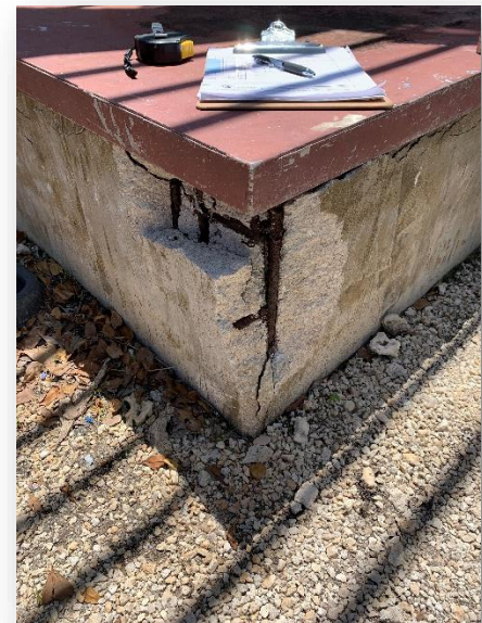
Collector tank damage at NW corner
