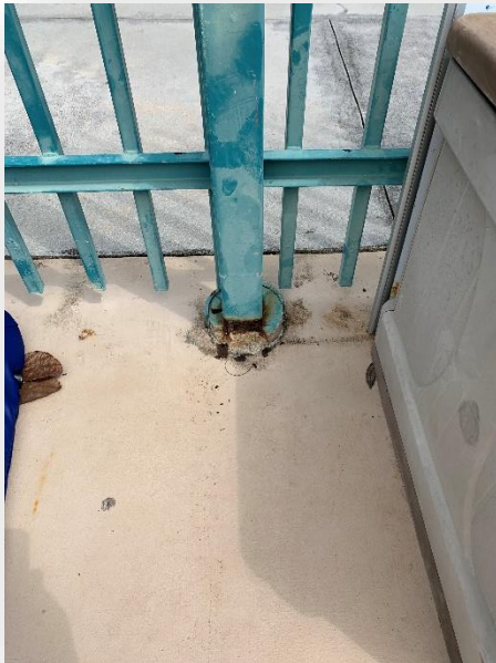
Corrosion of fence post on west side
