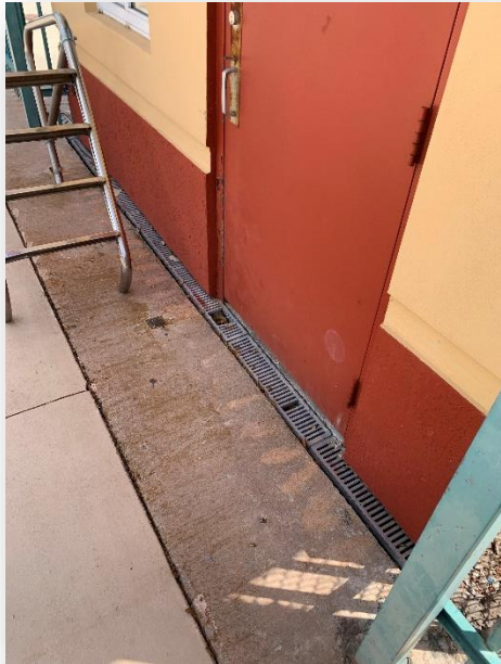
Deck drain settlement and separation at concession building
