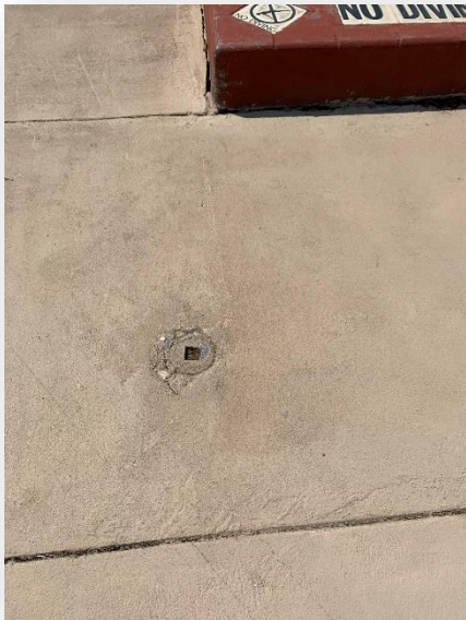
Spalling around cleanout in deck
