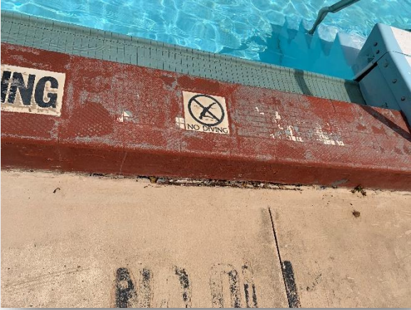
Settlement and deterioration of joint behind coping
