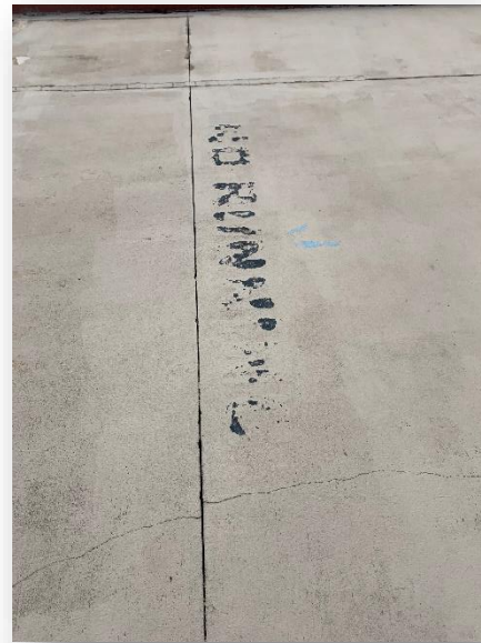
Cracking and distress in joint
