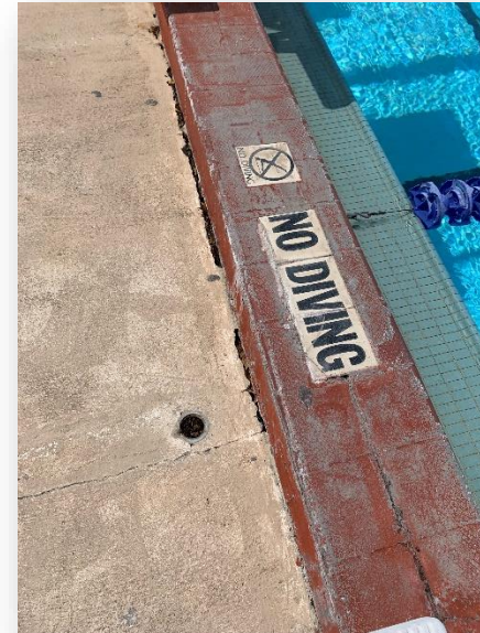
Distress and settlement behind gutter coping
