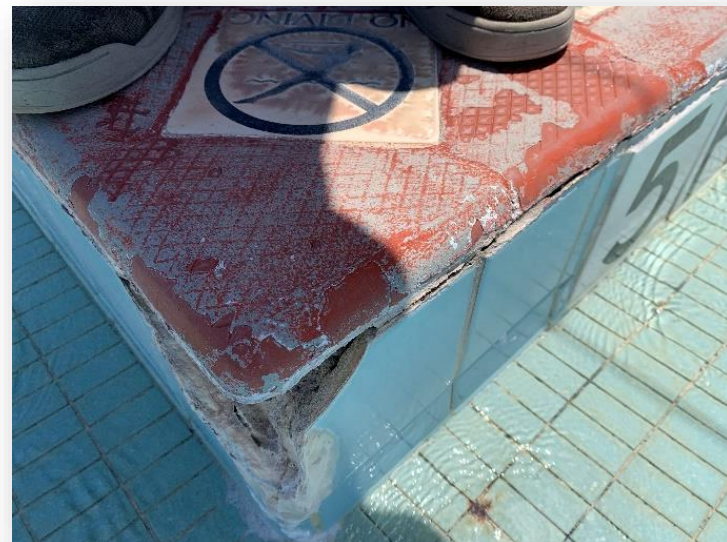
Damage and deterioration to pool and gutter corner
