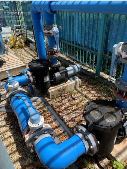
Pool pumps showing piping and control valves
