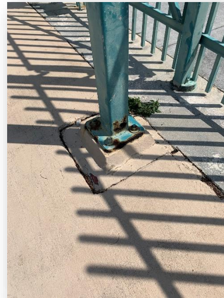
Light pole base showing corrosion in NE corner
