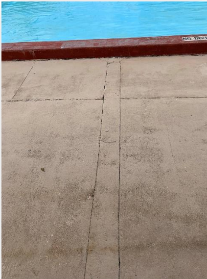
Crack in concrete repair
