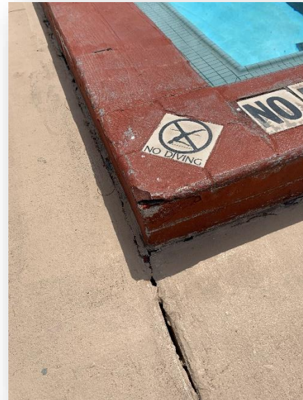
Damage to gutter coping and joint on southeast corner
