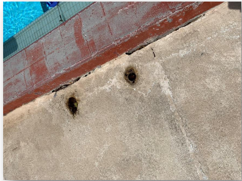
Old ladder inserts deteriorating in deck
