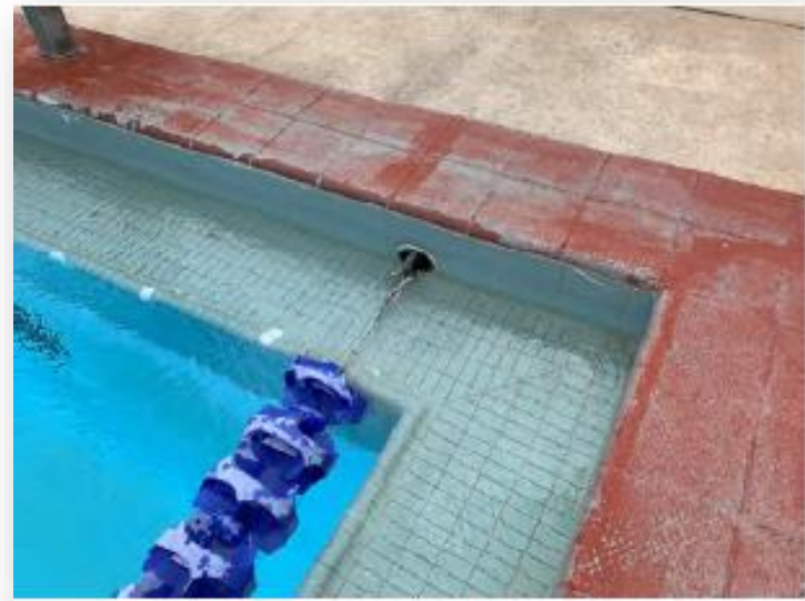
Gutter showing missing tiles
