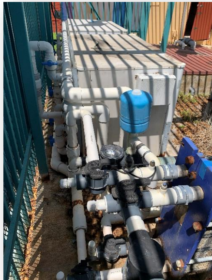
Geothermal heater units along with loop and well pumps
