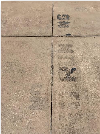
Lettering on deck fading and worn away
