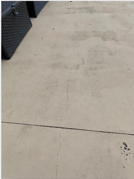
Cracking in deck near NW corner
