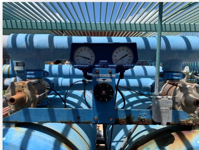
Filter controls showing corrosion on brackets
