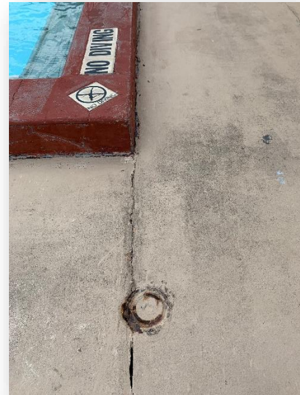
Old metal pipe embed corroding in deck at SW corner
