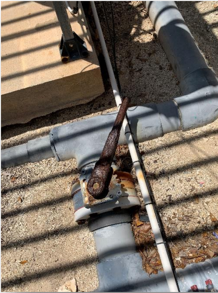
Master valve showing corrosion
