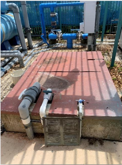
Collector tank showing infill lines and metal lid
