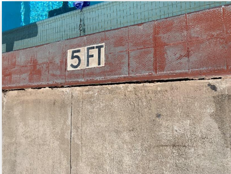
Settlement and loss of expansion joint material on east side
