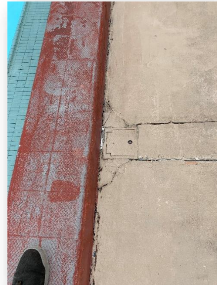
Distress and cracking at utility box on south
