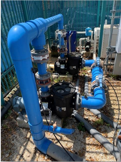
Pool Pumps with MCC, strainer baskets and piping
