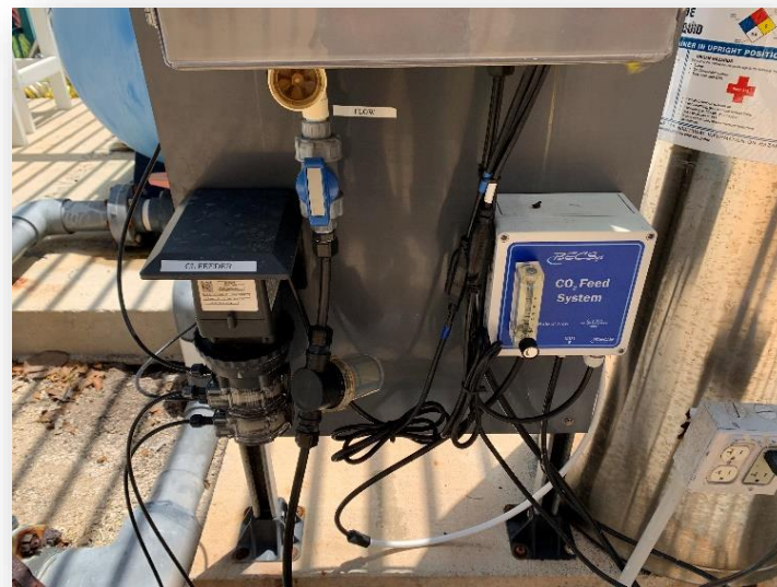
Chemical feed controls with chemical tubes.
