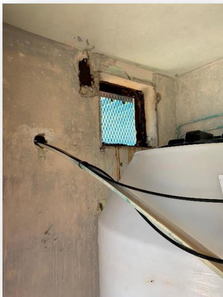
Corroded vent screen and metal in containment room
