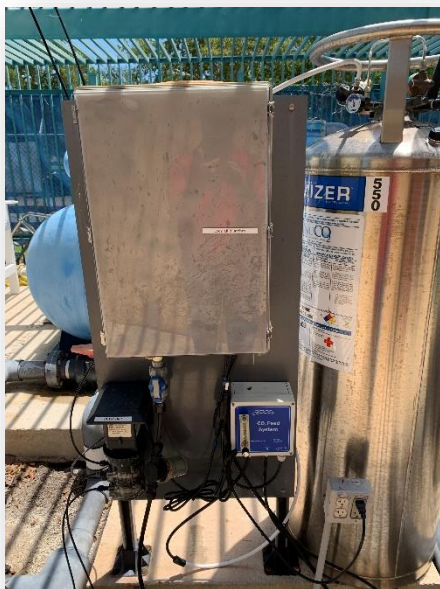
Chemical feed controls with CO2 tank
