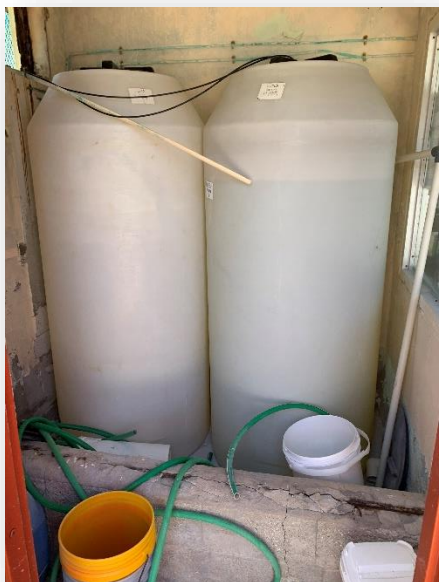
Chlorine tanks in Containment room
