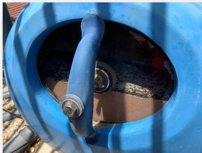
Filter window showing sand with debris
