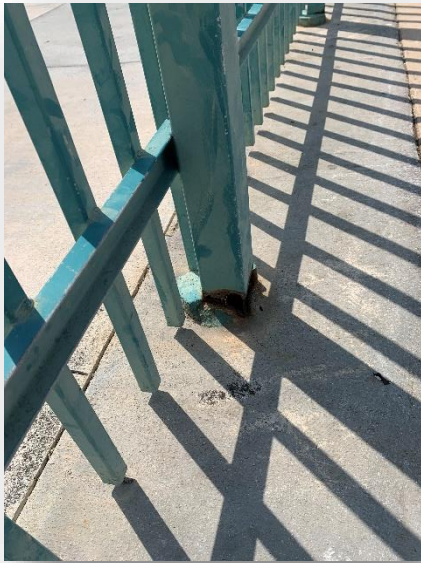
Corrosion of fence post on east side
