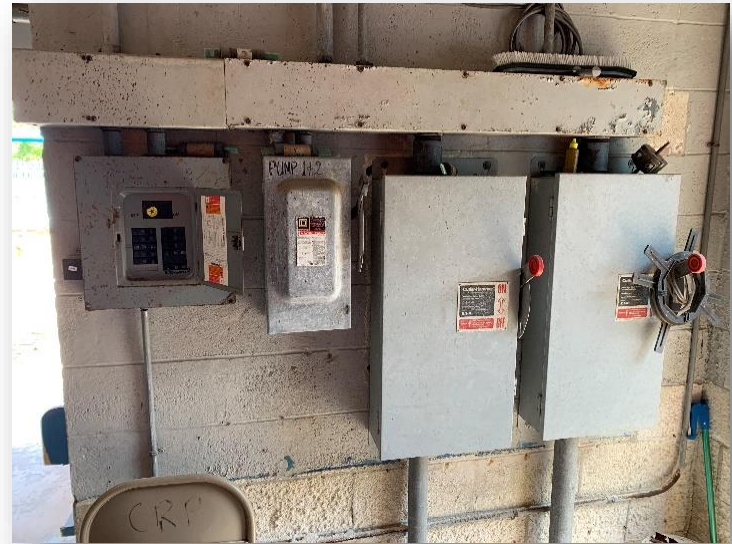
Electrical service—Two mains, pump controls and breaker
