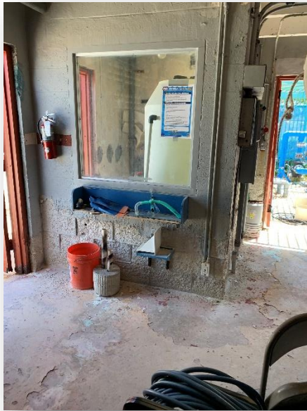
Containment room showing masonry block damage and floor delamination
