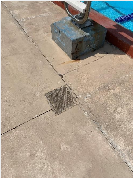
Distress and cracks around utility lid
