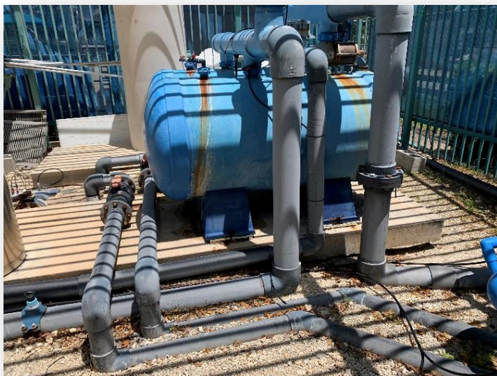
Filter piping—note rust on tank from blow off
