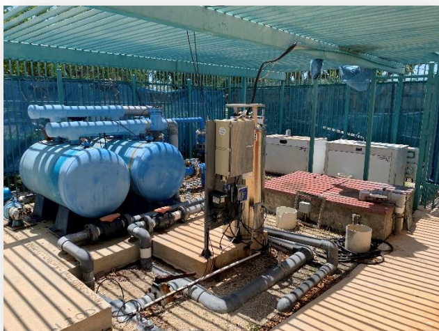
Equipment yard from NW corner—note chemical feed tubes along top
