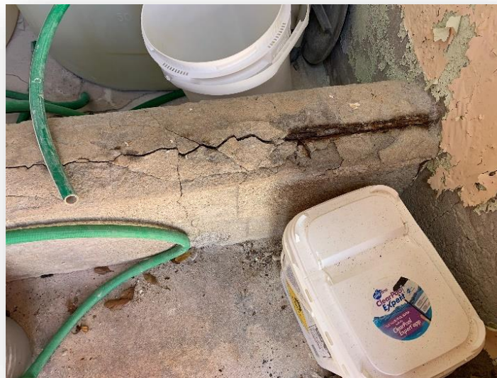
Cracked and corroded curb in containment room
