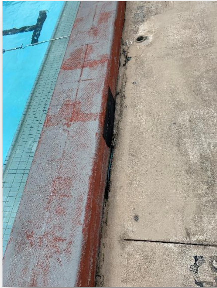
Loss of expansion joint material and exposed
