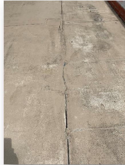
Reflection cracking on south side deck
