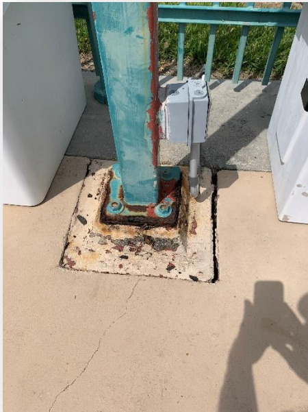
Light pole base showing corrosion in NW corner
