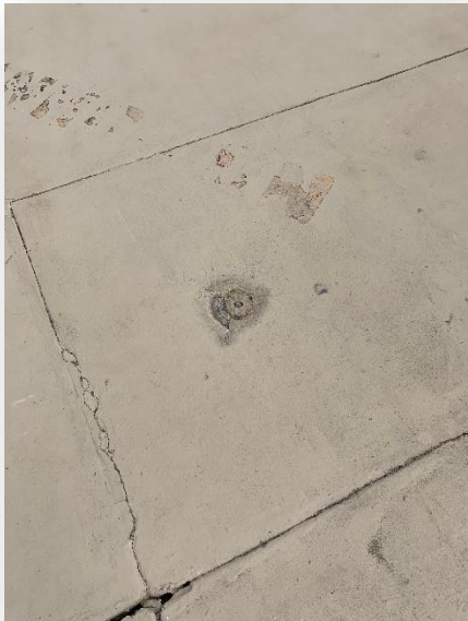
Cracking and distress around clean out in SW corner
