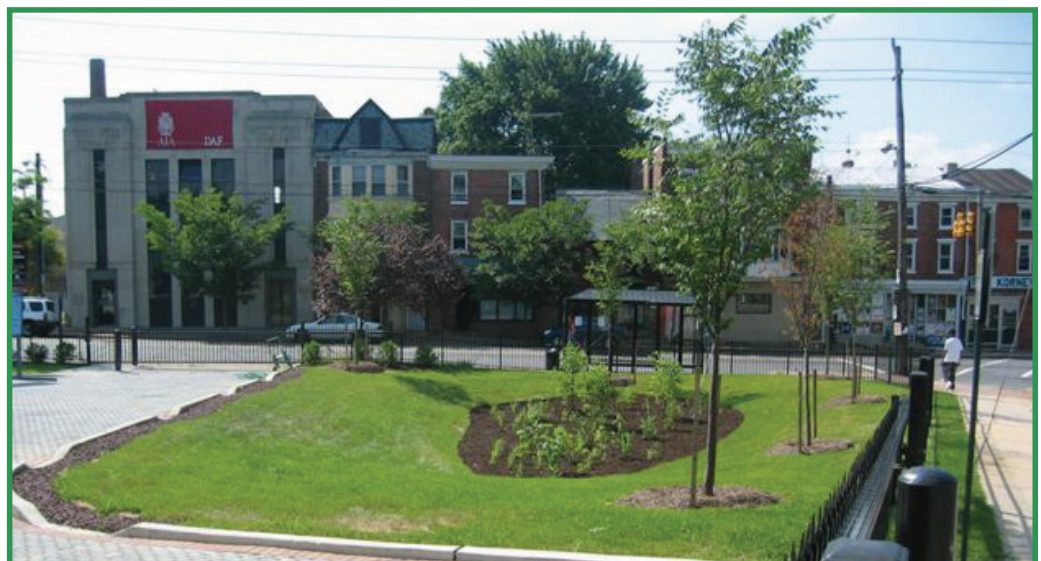
A bioswale in Wilmington, Delaware, designed to absorb and retain stormwater runoff.
